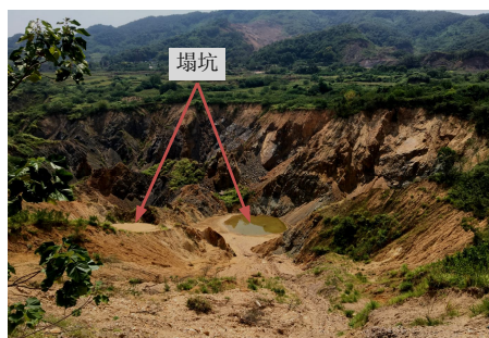
图 16 围岩蚀变带区域中的塌坑 Fig.16 Collapse crater in the surrounding rock alteration zone
